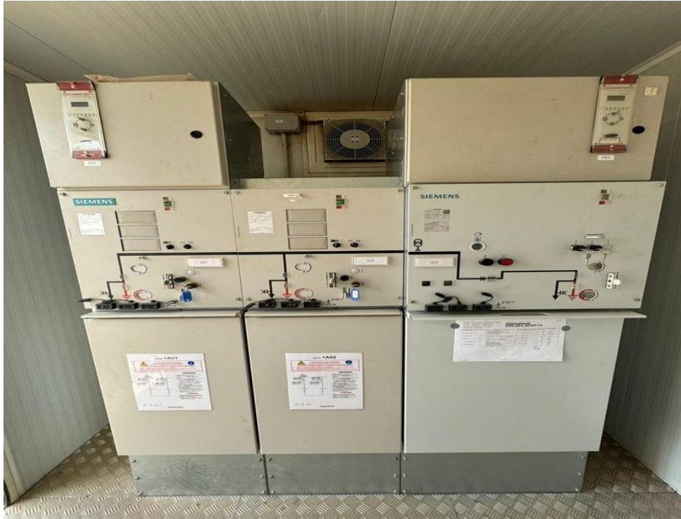
Figure 11 : Cellules HTA AO1, AO2, AO3
