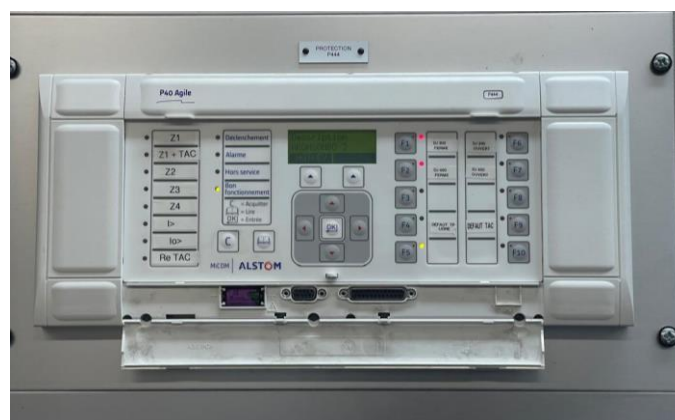
Figure 13 : Relais Micom P444
