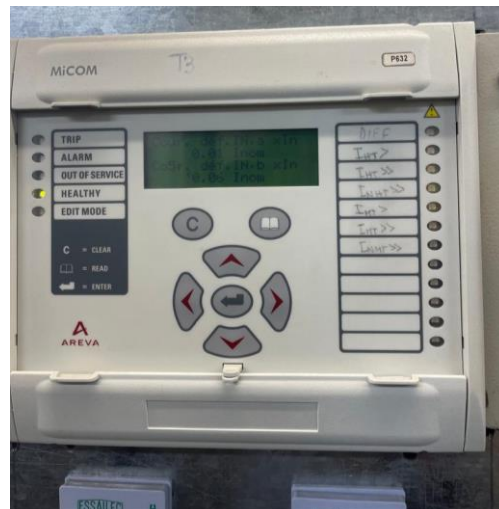
Figure 12 : Relais Micom P632
